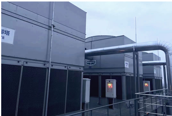
Plate heat exchangers and cooling tower for the cooling system
