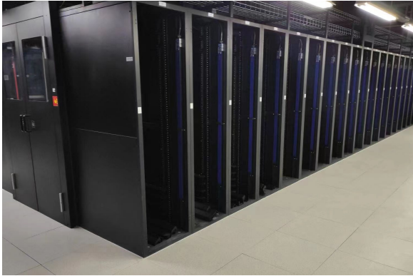
Cold aisle closure system
